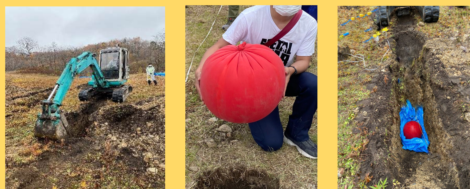
模擬空洞の作製 Reproduction of a Cavity
