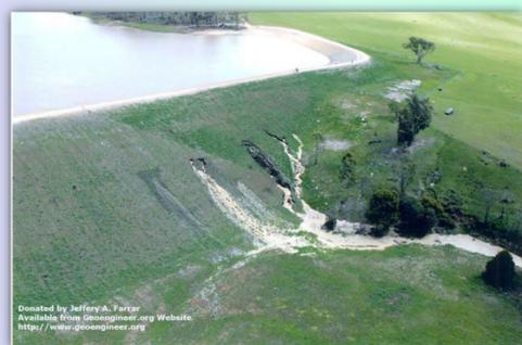
Internal erosion refers to the detachment of soil particles from the main soil structure due to the action of a fluid flow
