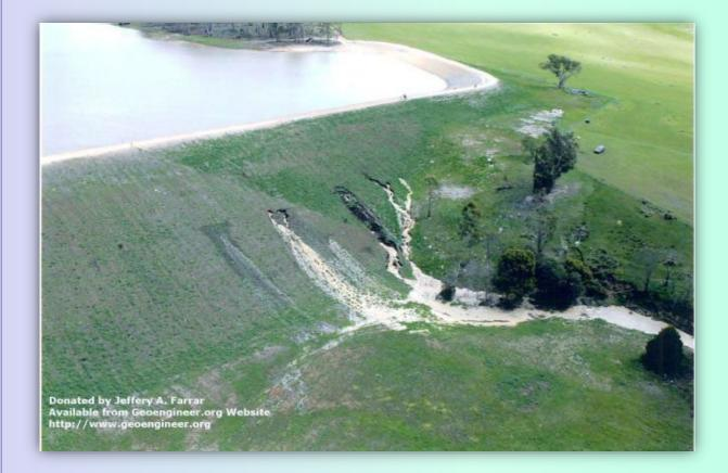
Internal erosion refers to the detachment of soil particles from the main soil structure due to the action of a fluid flow
