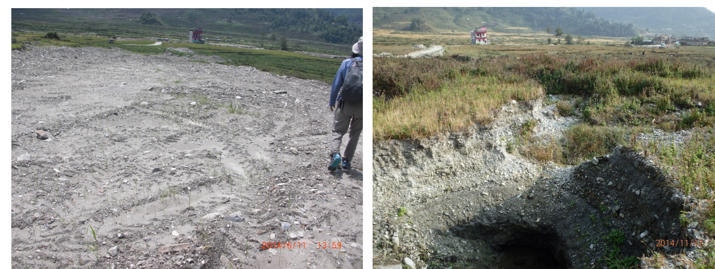
Photos taken from the same location (June 2014) (November 2014) 埋め戻された陥没孔の多くが雨季を経て再陥没 Refilled sinkholes had collapsed again after the rainy season
